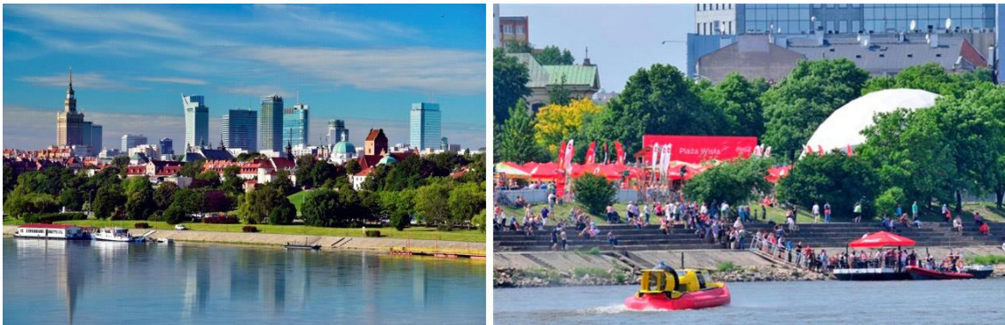
Figure 22. Embankment of the Vistula River. Warsaw, Poland.
