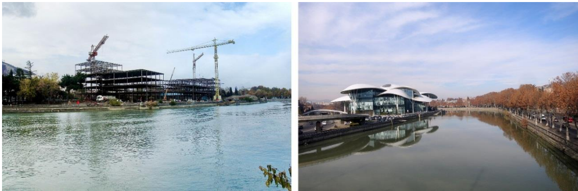
Figure 47. Construction Process and Finished Public Service Hall. Tbilisi, Georgia
