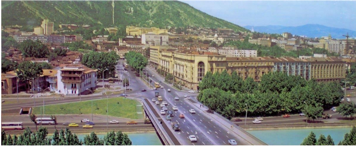
Figure 34. Baratashvili Bridge, Soviet Time. Tbilisi, Georgia. Source: National Parliamentary Library of Georgia
