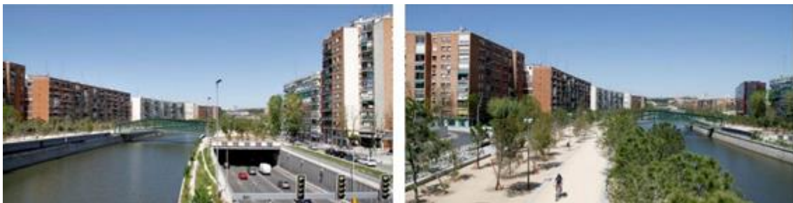
Figure 7. Tunnel and New Pedestrian Area of Madrid Rio Project.
