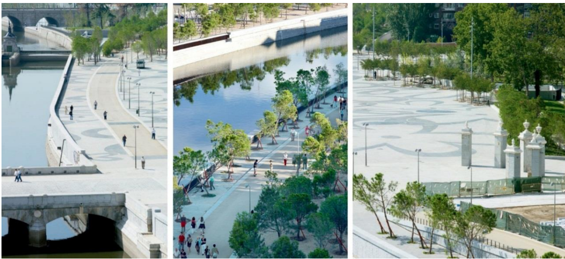
Figure 6. Embankments of Madrid Rio Project.
